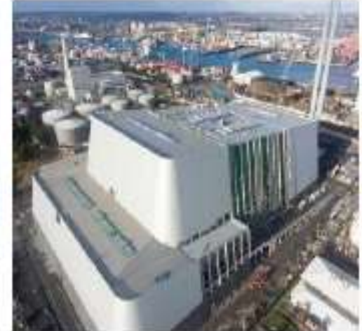
Dublin, Ireland – Covanta Energy
